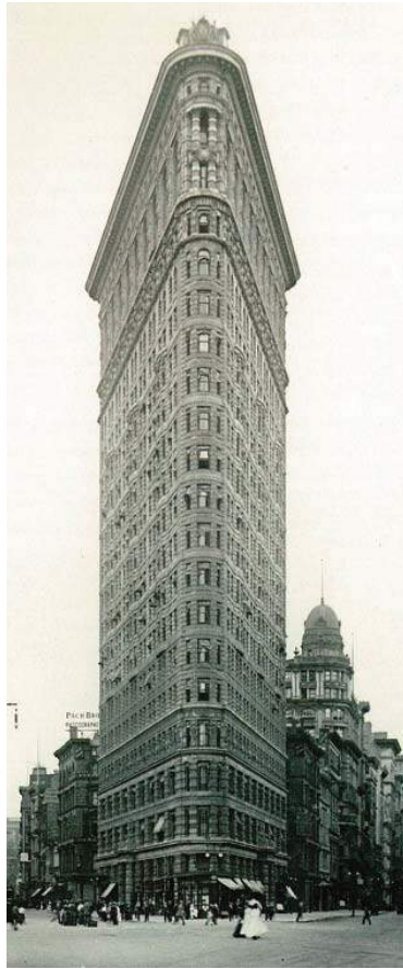
Historic Flatiron Building
